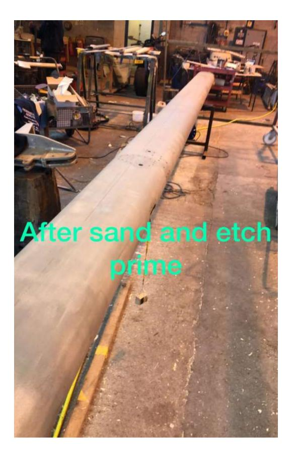
This is the mast that had to be stripped due to corrosion which led to the paintwork flaking and peeling off. First, I had to sand the old paint off mostly down to the bare metal so that the paint process could begin. I used an etch metal primer which was the first coat of paint that was put on. After the etch primer, another primer called light primer, as you can't paint topcoat directly over an etch primer.
