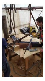
I also got to help build the Transom which taught me a new technique into connecting wood and give me good experience in joinery work. The Transom was then also painted with red oxide to ensure that it stayed clear from the elements.
