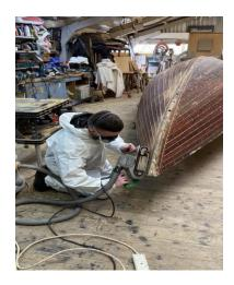
Once the glue had hardened overnight, I began removing all the staples I had previously left in the veneers with a small flat bladed screwdriver and a pair of pliers. After I had finished removing all of the staples I carefully went over the repair with a block plane to remove any
